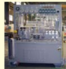
River Gate Unit
