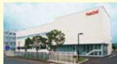
Eastern Japan Service Center (Ayase City, Kanagawa)
