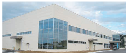
Hydraulic motor factory (increasing production capacity)
